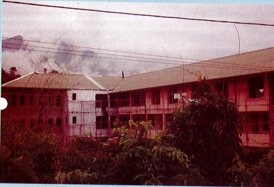
Construction of the Faculty Building of Social Sciences and Languages
