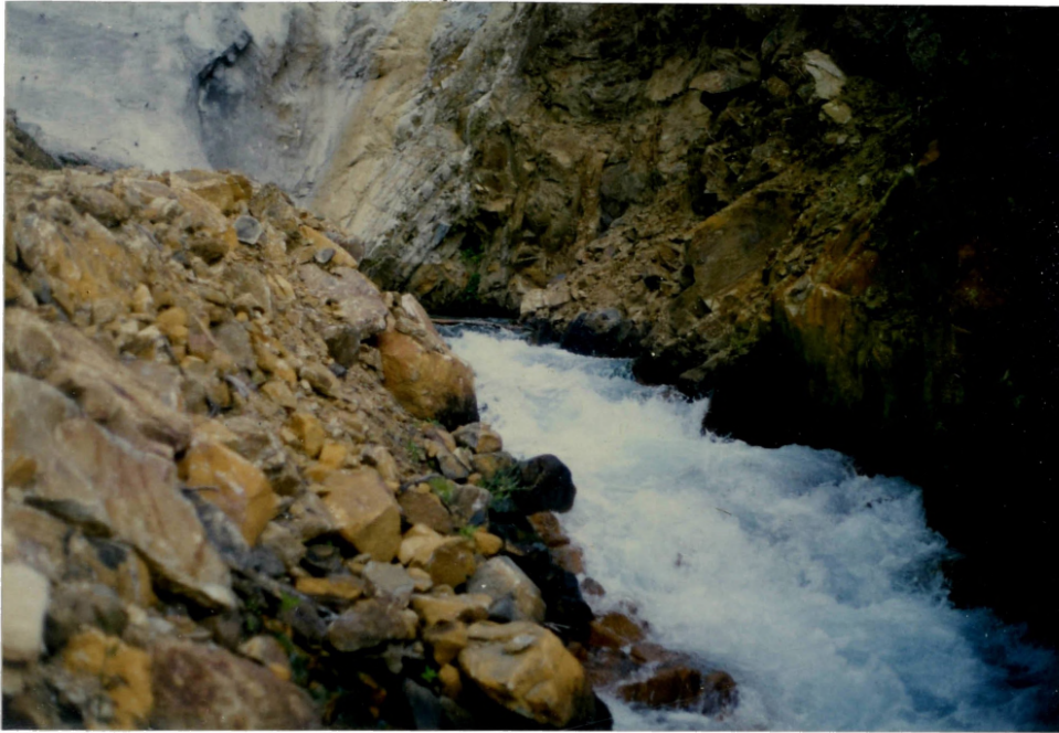
Plate 1: Leakage Point at Matihakka
