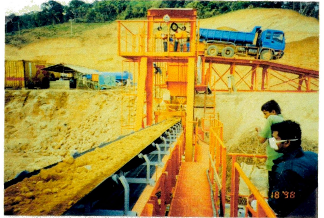
Loading of Material by Belt Conveyor
