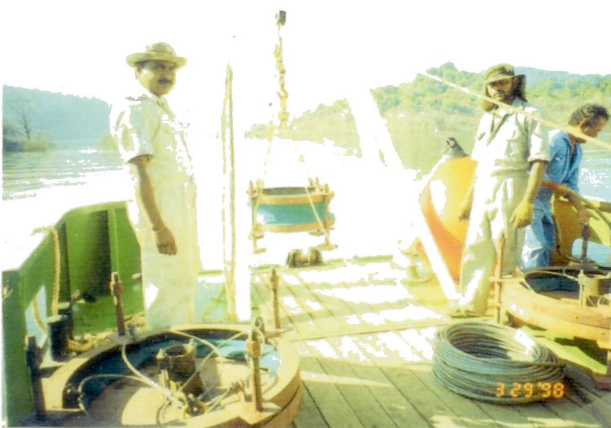
Placing of Disturbed Sampling Tray
