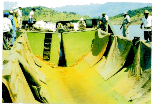
End of Complete Operation after Taking-Out of Canvas Sheets
