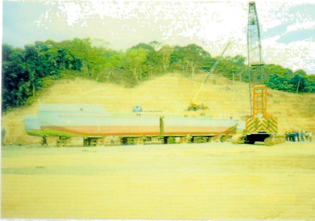
Assembling Works of No. 1 and No.2 Barges (28.02-13.03.98)
