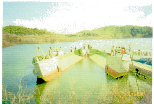
Coupling of Two Half Hulls of No.1 Barge (15.03.98)
