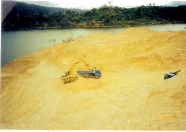
Developing of Pilipota Borrow Site
