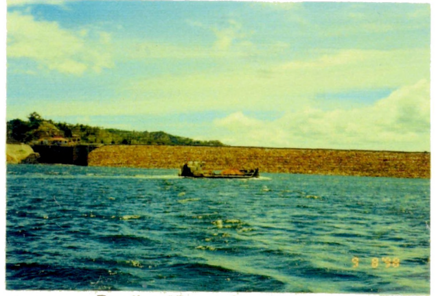
Traveling of Barge to Dumping Area
