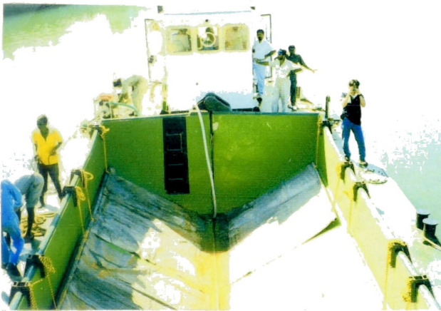
Dewatering of Barge Hopper after Arrangement of Canvas Sheets
