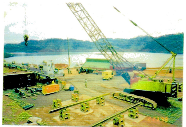
Delivered 1 st Piece of Barge to Site on 23.02.98
