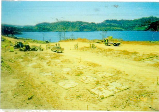
Completed Concrete Foundations of Assembling Yard on 31.01.98
