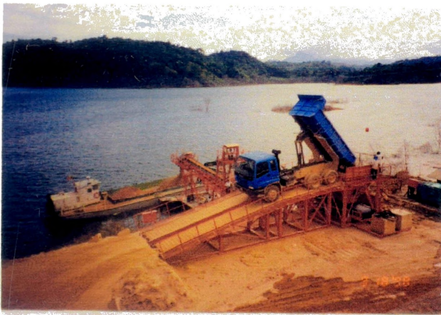
Access Ramp to A Hopper for Dump Truck
