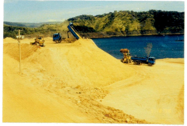
Stockpile Yard at Kinchigune
