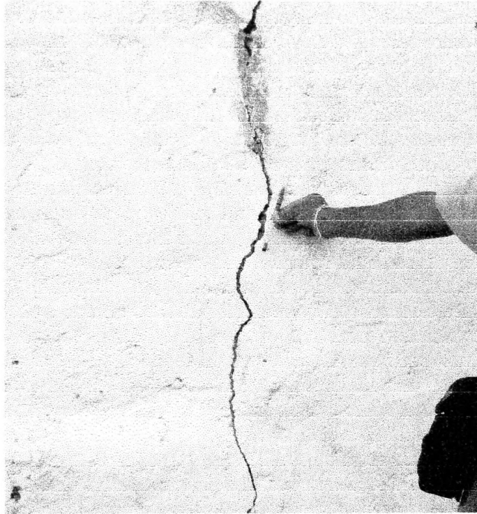
Plate 4.3 :- A fracture observed on the wall of a line cottage
