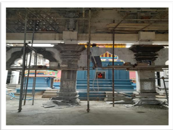
Fig 2: Construction work is going on inside the Kannagi Amman Temple
